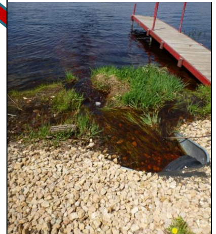
Cty Rd K Culvert
